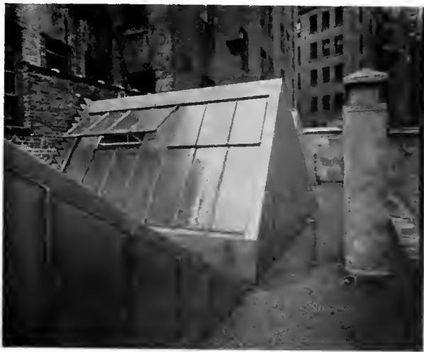
SAW-TOOTH ROOF WHICH REPLACED OLD SKYLIGHTS
